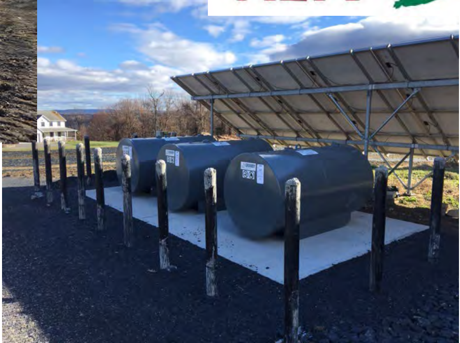
3 On Farm Secondary Containment Facilities
