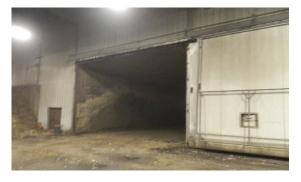
The in-vessel composting process is similar to covered aerated static pile composting in that the piles are aerated continuously (with a combination of positive and negative air flow) and contained in a vessel. The difference is that the piles are contained in a rigid structure. The vessels are made of concrete, with gasketed and insulated stainless steel doors. The residence time for this type of system is in the order of 28 days with several additional weeks
