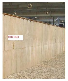
*Photo 8 – RTD temperature sensor mounted in bay wall box.*  The temperature inputs from the same aeration zone in each of the five (5) bays are averaged by the control system to drive the blower drawing air from the respective zone. All blowers are operated through a variable frequency drive (VFD) to provide continuous modulation of the air flow to precisely maintain process material temperature about a floating set point within the control system.
