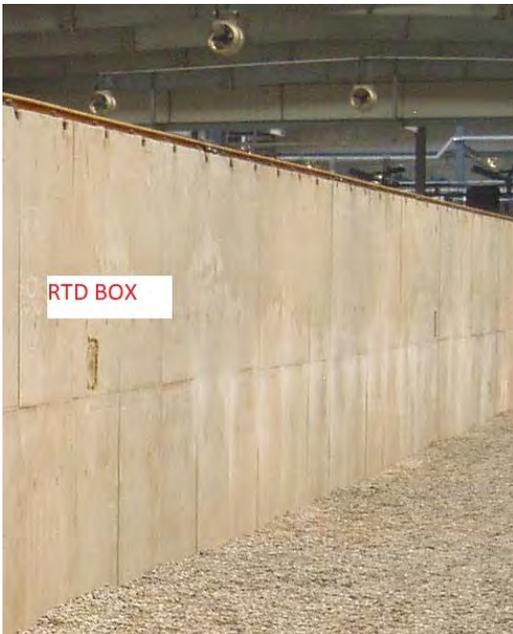
*Photo 8 – RTD temperature sensor mounted in bay wall box.*
