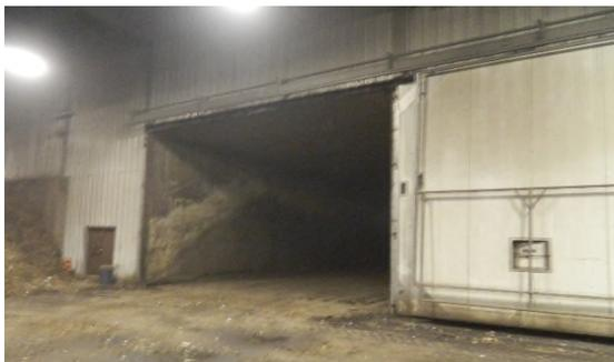
The in-vessel composting process is similar to covered aerated static pile composting in that the piles are aerated continuously (with a combination of positive and negative air flow) and contained in a vessel. The difference is that the piles are contained in a rigid structure. The vessels are made of concrete, with gasketed and insulated stainless steel doors. The residence time for this type of system is in the order of 28 days with several additional weeks
