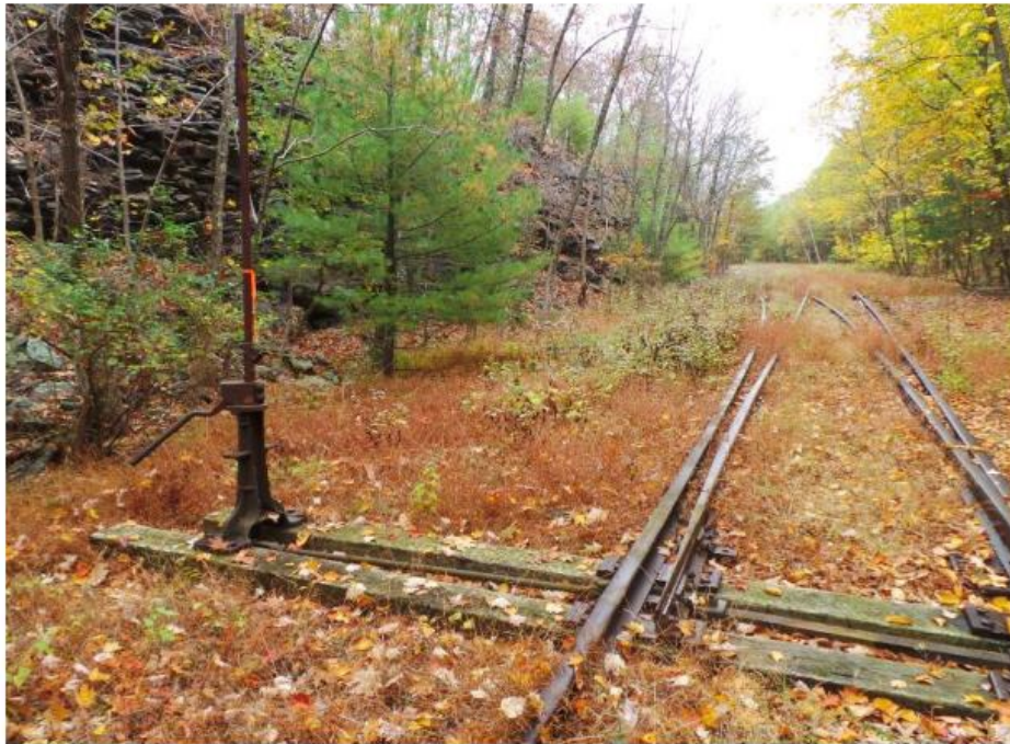
Photo 1-1 – Example of Remaining Railroad Track Infrastructure – Segment 1
