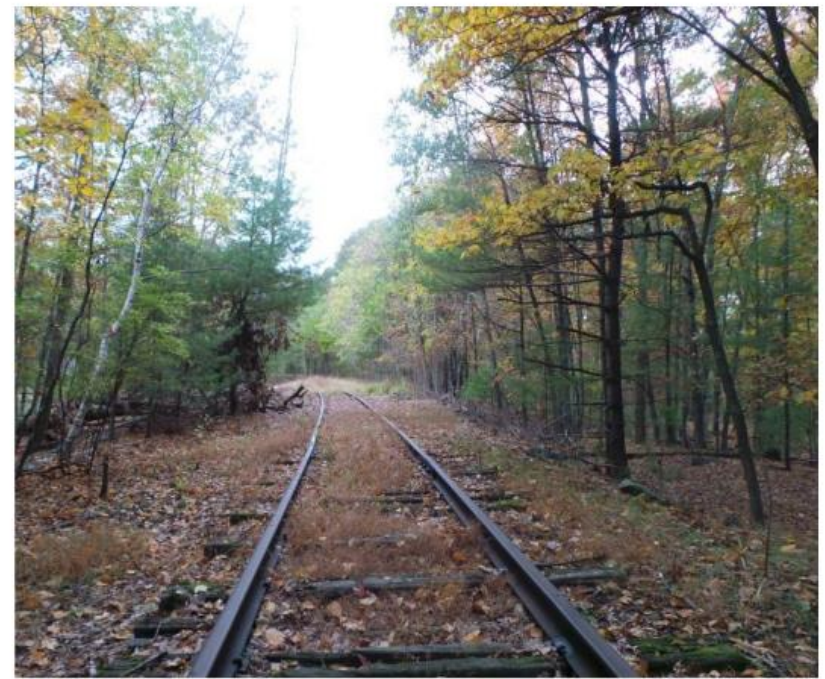
Photo 1-2 – Existing Rail Infrastructure Conditions – Segment 1
