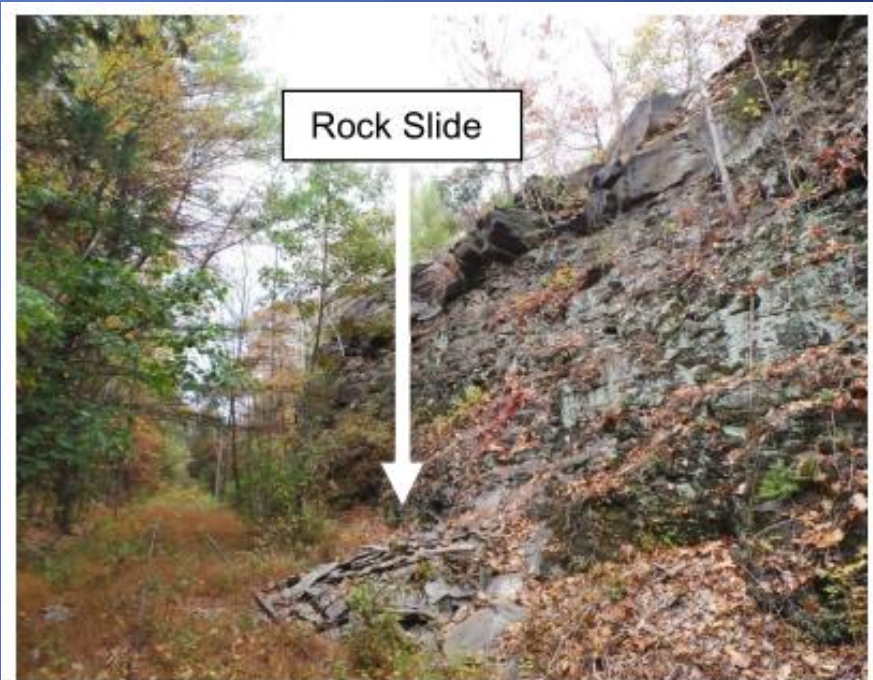
Photo 1-5 Rock Slide in Segment 1
