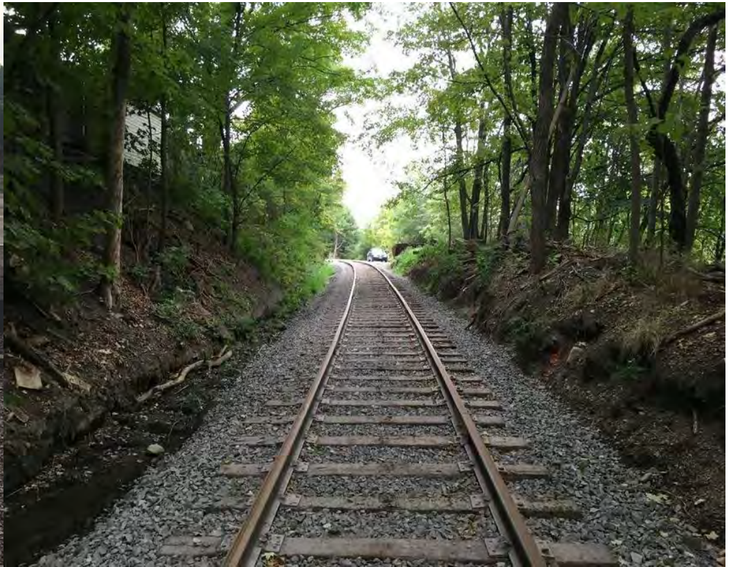
Track Reconstruction at MP 6.2
